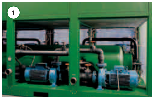
1. Stand-by pump. Bomba en stand-by. Stand-by Pumpe.
